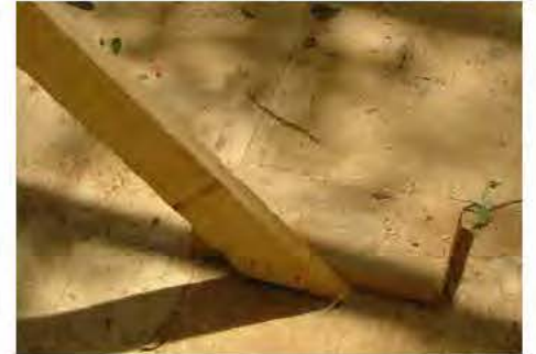
Figure 2. Nail your bracing to a block that is nailed to a joist.
