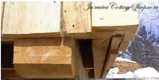
Bottom of building showing 4x6 skid placement and bottom of siding and trim
