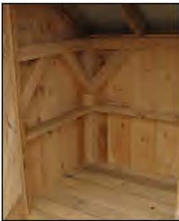
Figure 8-Angle Bracing
