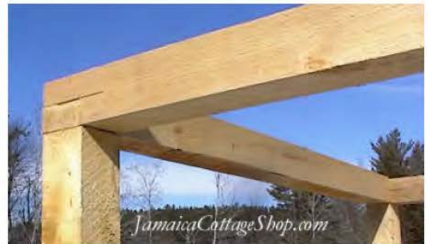
1/2 lap 4x4 top plate corner attachment
